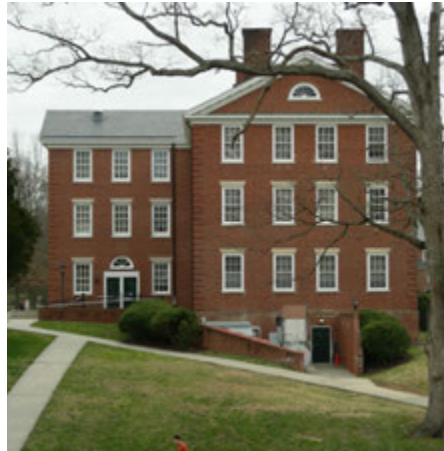
Morton, North Façade
