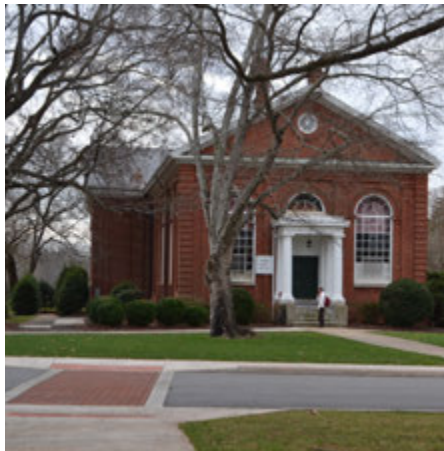
Winston Hall, North Façade
