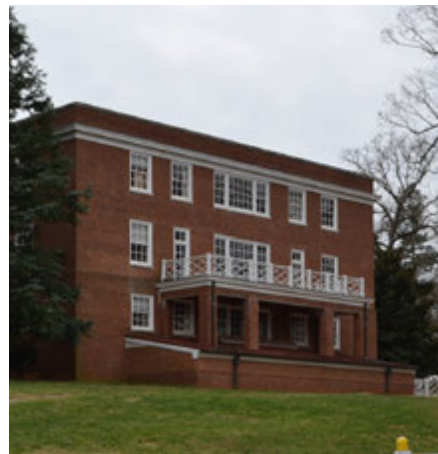
Eggleston, North Façade
